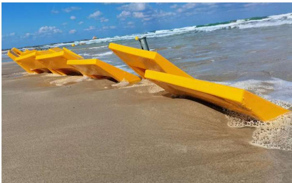
> The modular system aims to keep the sand on the shoreline, which would otherwise be dragged and dispersed into the sea due to run-off.
